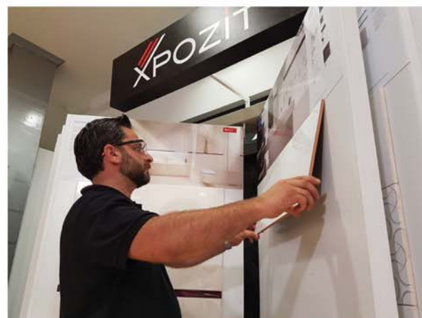
ADD THE FIRST CERAMIC TILE AND CAREFULLY CENTER IT
