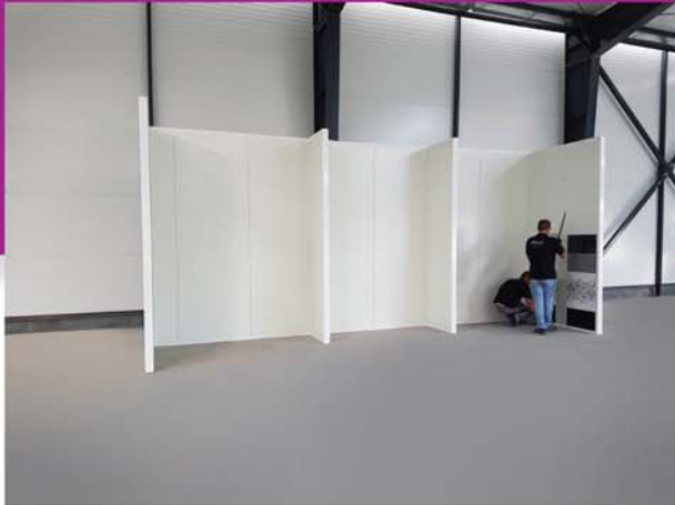
Booth being completed, workers will start to install the magnetic tiles
