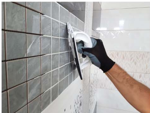
After the tiles are completely installed, plaster is applied. The system allows the plaster application and easy removal without leaving marks, whenever a tile change is required.
